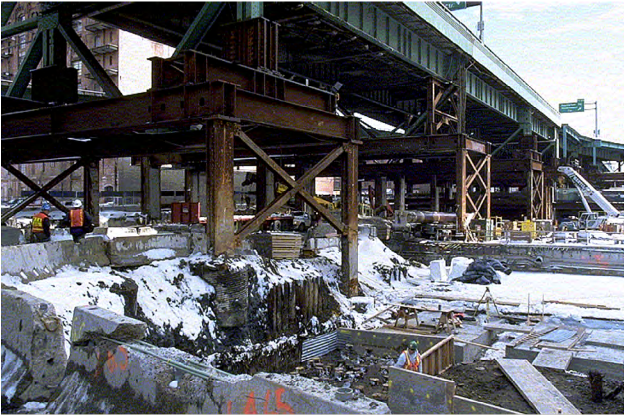
Figure 30: Underpinning of Existing Viaduct – Central Artery Tunnel Project in Boston
