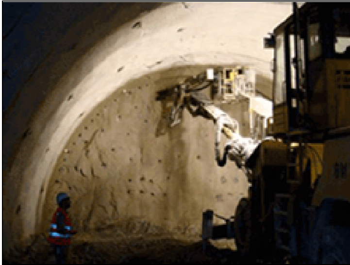
Figure 45: Drill and Blast Operations (SEM Tunneling)
