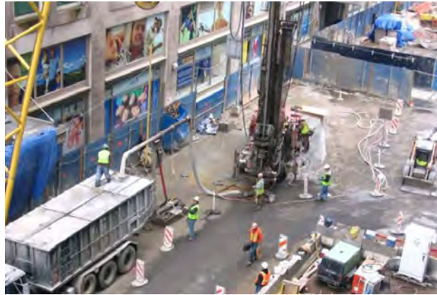
Figure 32: Jet grouting ground improvements for North Shore Connector
