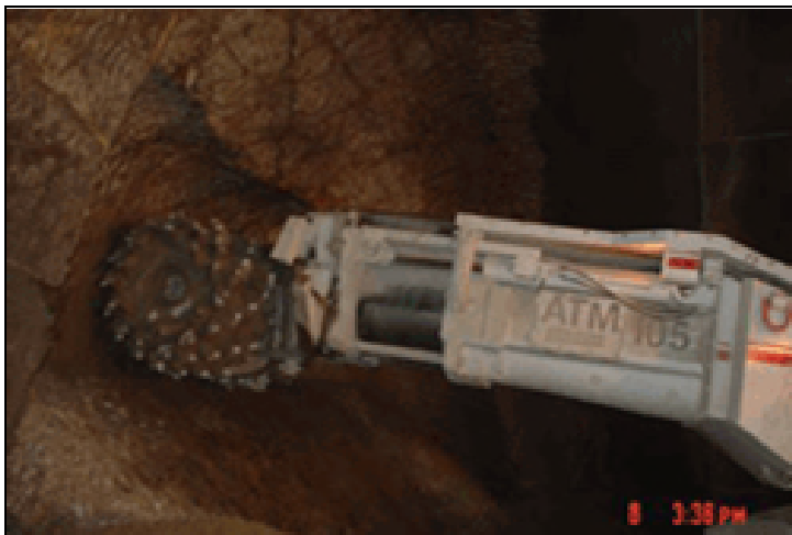
Figure 46: Tunneling with a Roadheader (SEM Tunneling)
