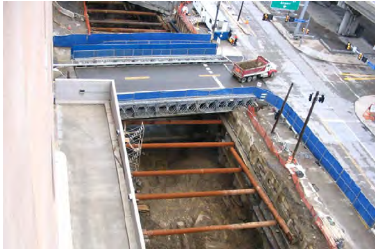
Figure 26: Temporary Access at Roadway Crossing for Pittsburgh North Shore Connector
